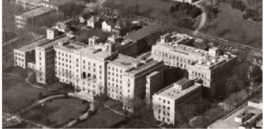
Among the buildings behind Wisconsin General Hospital (now called the Medical Sciences Center) is UW Children’s Hospital (now called the Bradley Building), where Fritz Bach, MD, performed the first successful bone marrow transplant in 1968.
